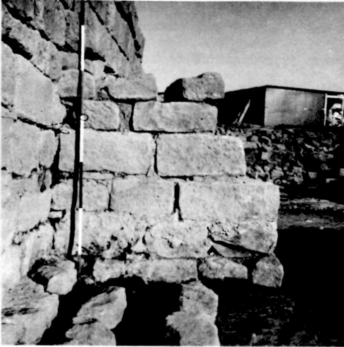
Fig. 20. Photograph of counterfort # 3, looking E .
